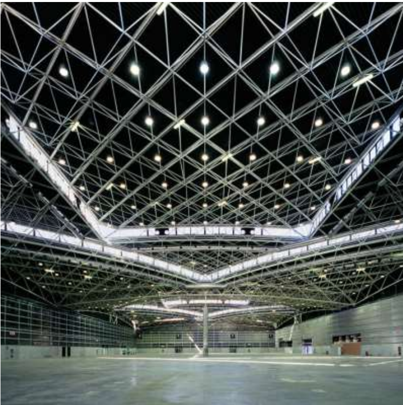
Pavilion 1 and Pavilion 2 - Internal view
