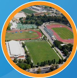
UNIVERSITY STADIUM OF LISBON
